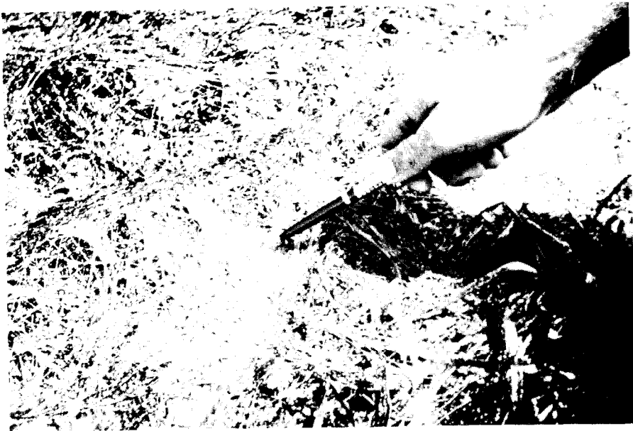
Figure 17. Fiber Glass Roving and Asphalt Cement Two Applications
