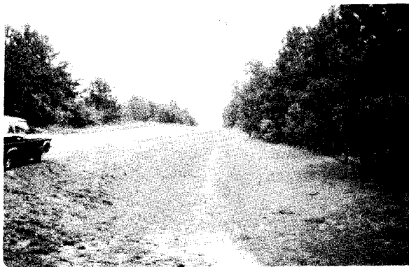
Figure B-9 Test Channel No. 3-FGR after permanent grass liner had been established. This picture was made two months after Figure 9.
