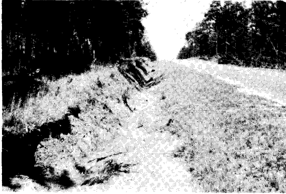
Figure B-2 Test Channel No. 1-FGR before reworking.
