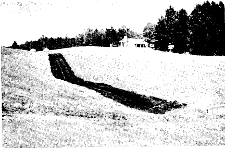
Figure 21. Roadside Drainage Channel Lined with Two Applications of Fiber Glass Roving and Asphalt Cement
